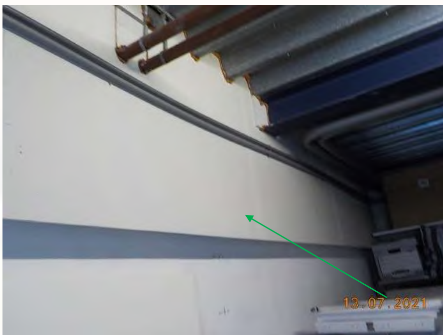
Foto 6: Bron B02, Asbestvrije beplating, brandwering
